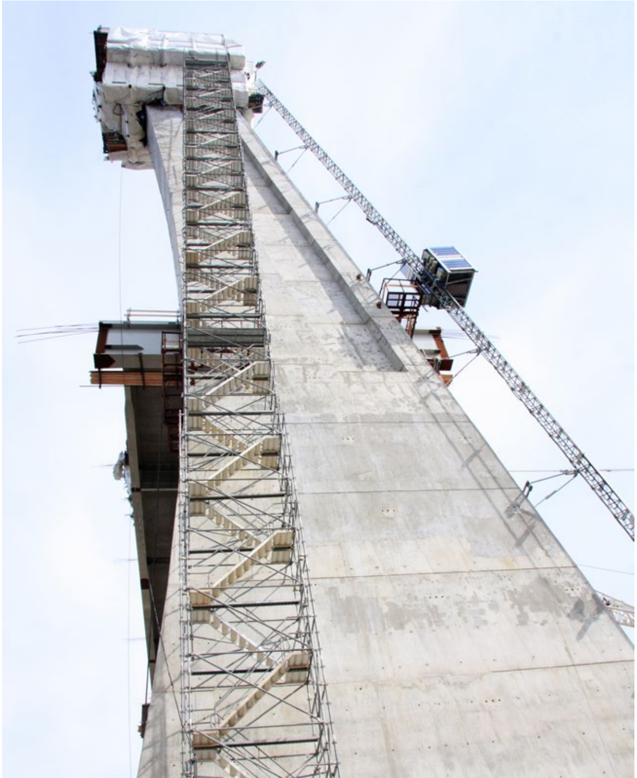
Scaffolding and surface protection work on a bridge construction in St. Petersburg, Russia
