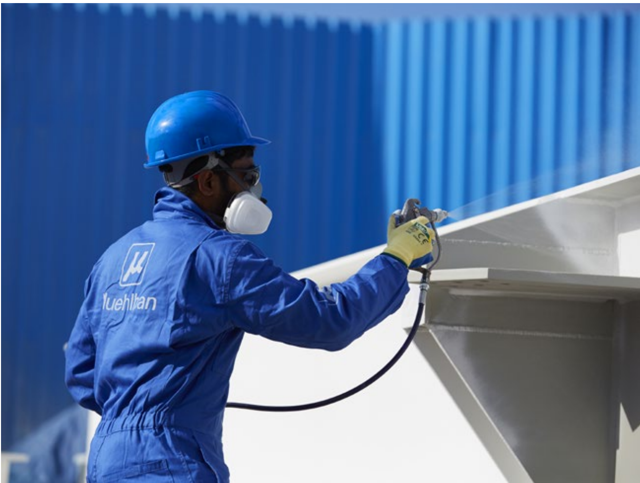
Fire protection coating
